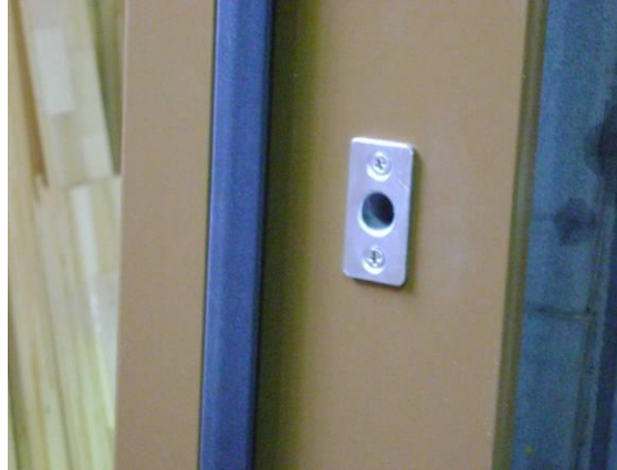
Fig-4 Wall Pivot socket
